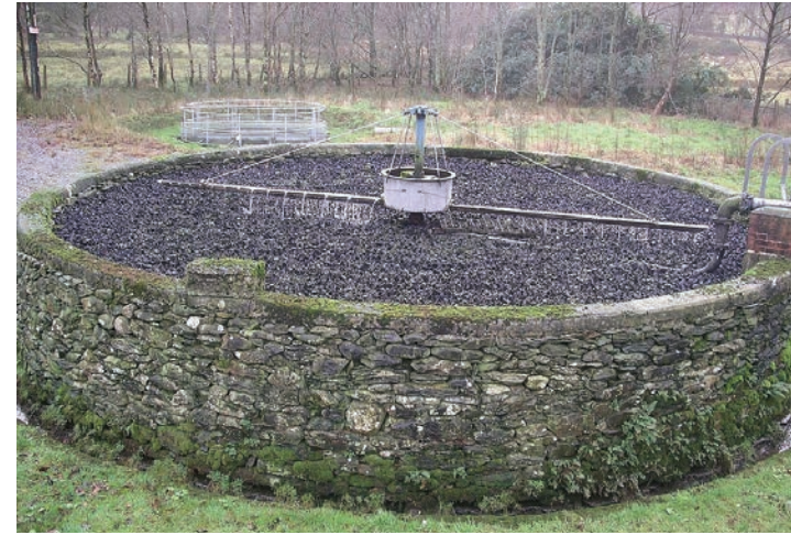
(Top) Example of Trickling Filter Bed (Bottom) Dye Trace from School Restroom to Sequiota Spring
