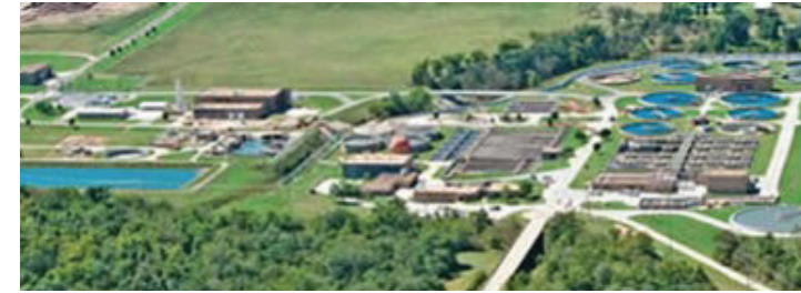
Springfield Southwest Wastewater Treatment Plant
